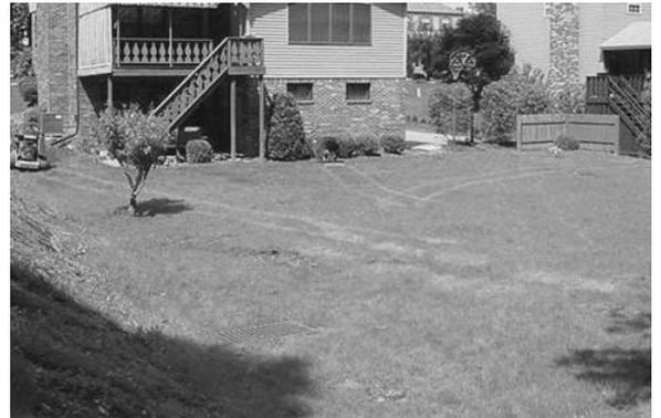
*The slope of this backyard caused water to sit for weeks, which can lead to problems for the foundation.*
